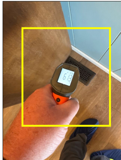
The differences in air temperature measured at supply and return registers fell within the acceptable range of between 14 and 22 degrees F.
